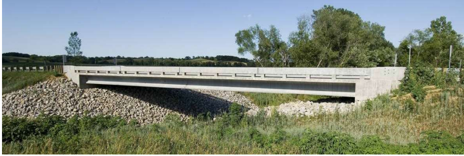
Figure 5. Mars Hill Bridge, Iowa, USA (2006) [20]
